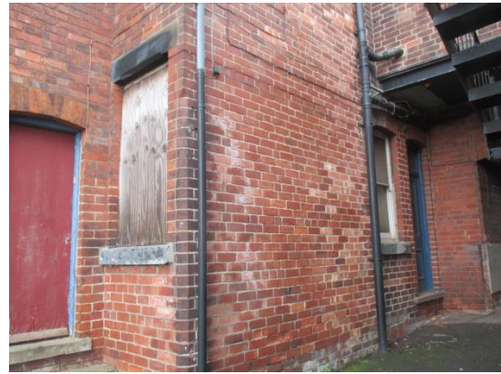
Detail of 248 Derby Road
