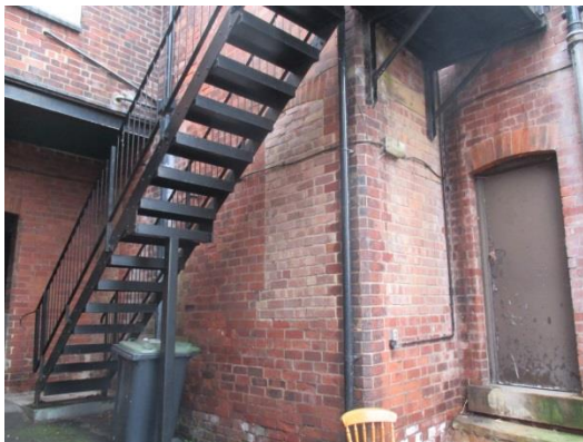
Rear of 250, former window openings
