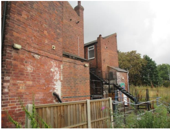
Wider view of 250 to 254 Derby Road
